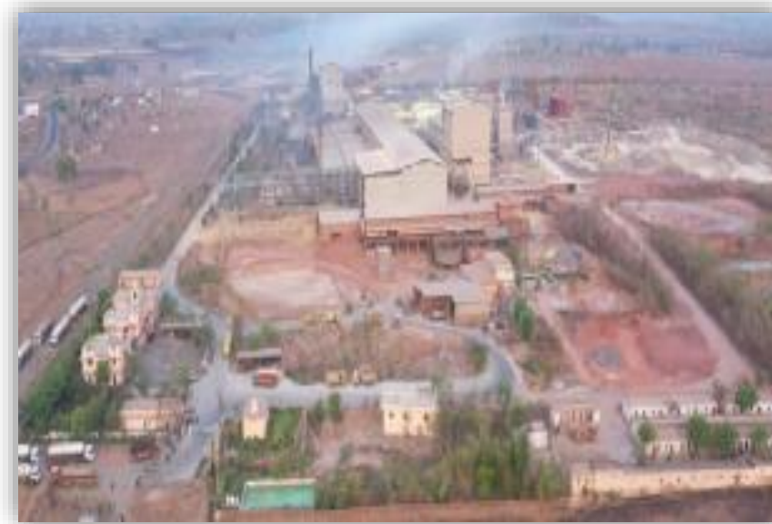
Banda Plant in Sagar
